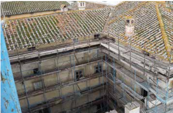
In this photo: The state of deterioration of the roofs before restoration
