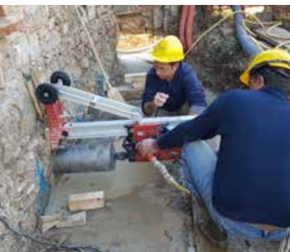
In this photo: Coring through masonry
