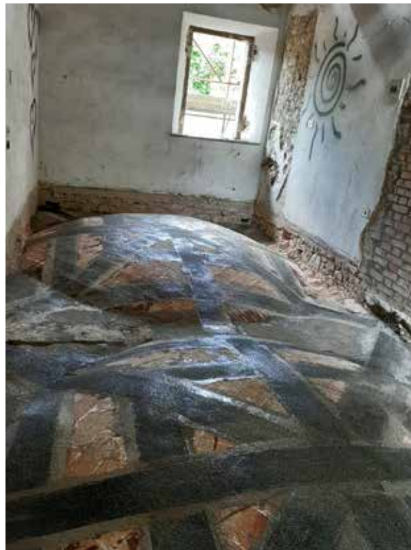
In this photo: Consolidation of a vault with carbon fibre bands.
