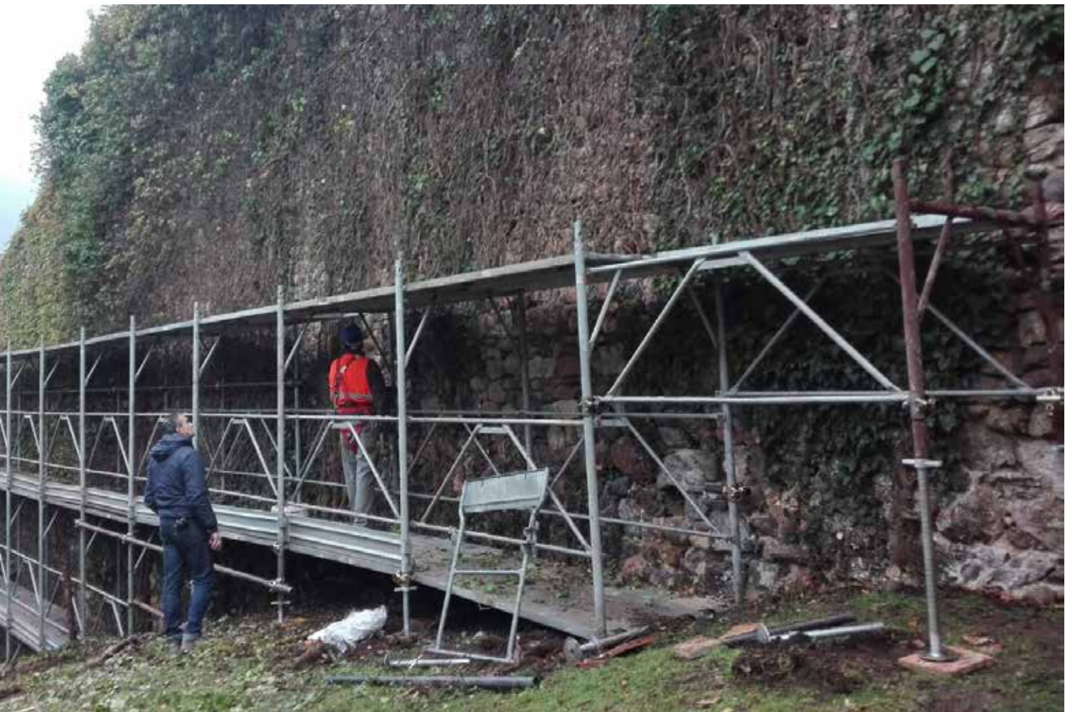
In this photo: Erection of scaffolding
