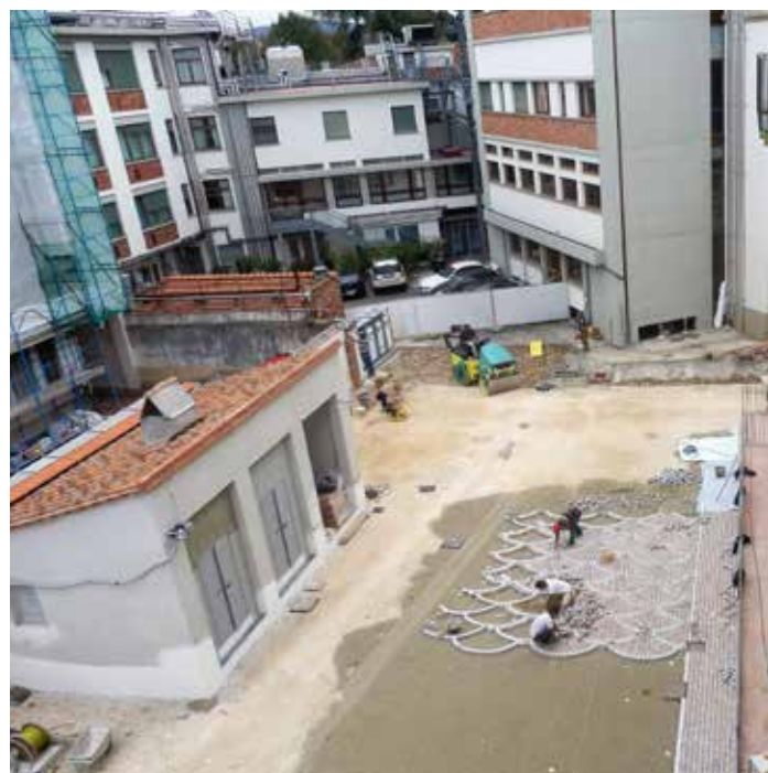
In this photo: Construction of the external porphyry floor
